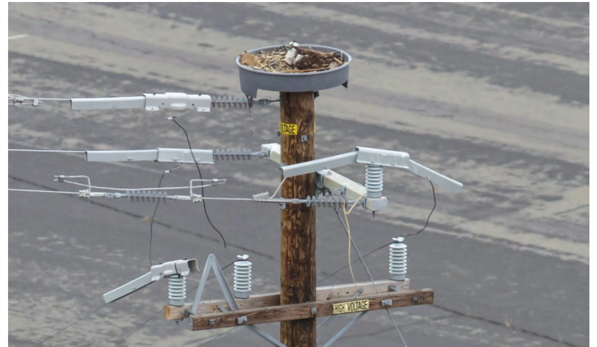
Osprey nest on power pole in Rodeo; This nest was seen to have collapsed on June 11, 2013 (upper photo). Pacific Gas & Electric workers added an artificial nest structure and modified the wiring later that year. In each subsequent year, it has hosted an active Osprey nest. Photos: Anthony Brake
